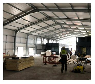
sandwich a PIR insulation. That is available in depths of 40mm, 60mm, 80mm, 100mm and 115mm. If you are just looking for an insulated building, to only be used for a limited time each day. The 40mm depth panel is ideal, if you plan on having people working in the building for long periods. The normal go to depth, is 115mm for the roof sheets and 80mm for the wall sheets. This will generally meet the Part L requirement for the external skin. If the building is to have a permanent heat source.
